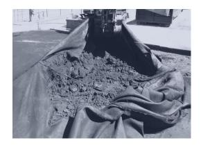
CTP environnement suggested implementing a costeffective solution in terms of mechanical equipment, which was quick and easy to set up. Dewatering using the Geofloc® process combined with geotextile membranes has indeed various advantages:
